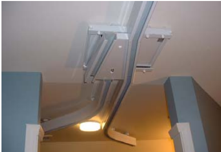
Powered by the hoist, both the electric turntable and exchanger are easily installed and allow an endless variation of options.
