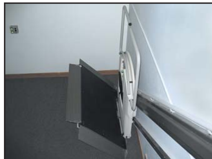
The Auto Fold feature automatically folds the platform if left unattended for a period of time at a landing (optional)
